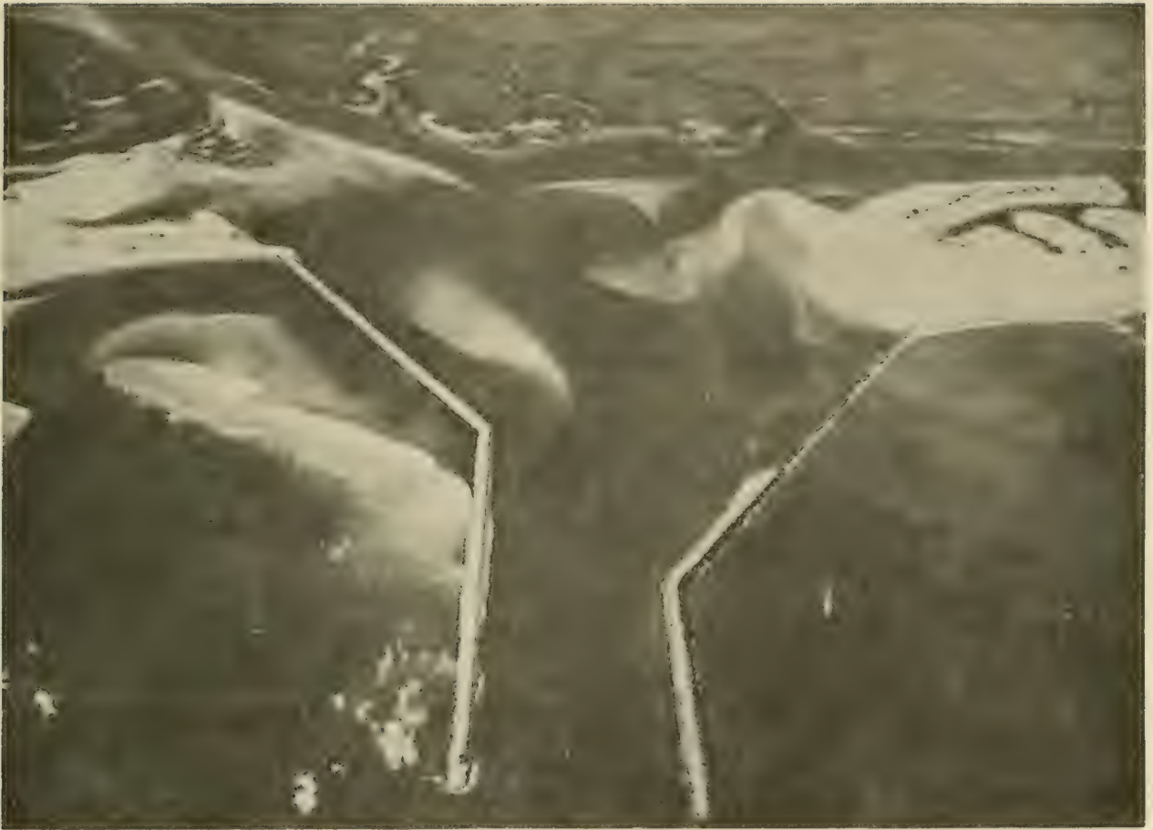
Figure 1-13. Weir jetty at Murrells Inlet, South Carolina, 1981.
