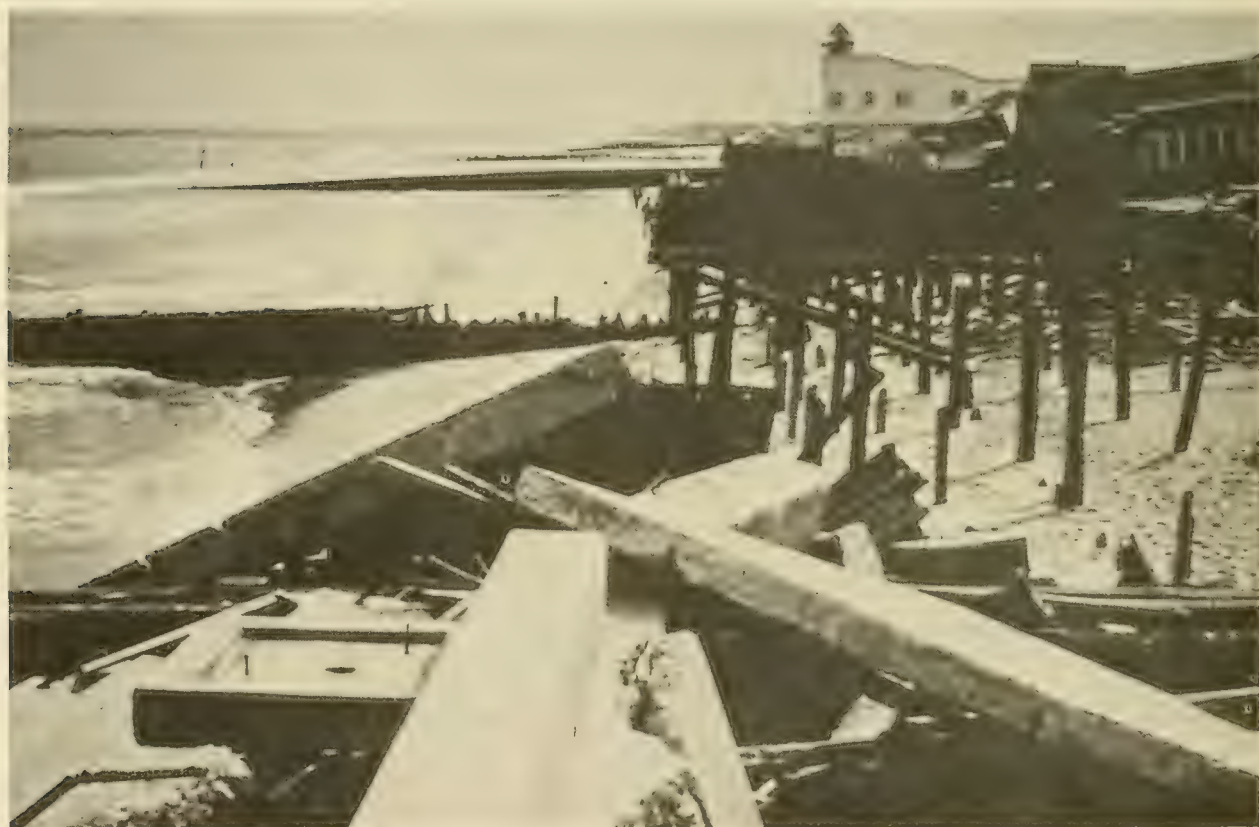
Figure 1-10. Damage after the 1962 storm, Rehoboth Beach, Delaware.
