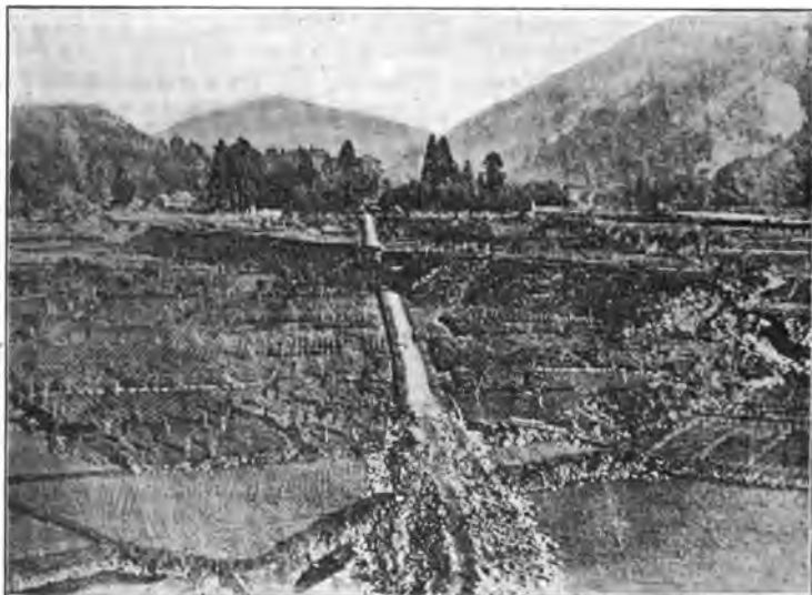
FIG. 7.— Fault-scarp in the Neo Valley, Japan, earthquake of 1891. The road shows a slight horizontal as well as vertical displacement. (Milne)
