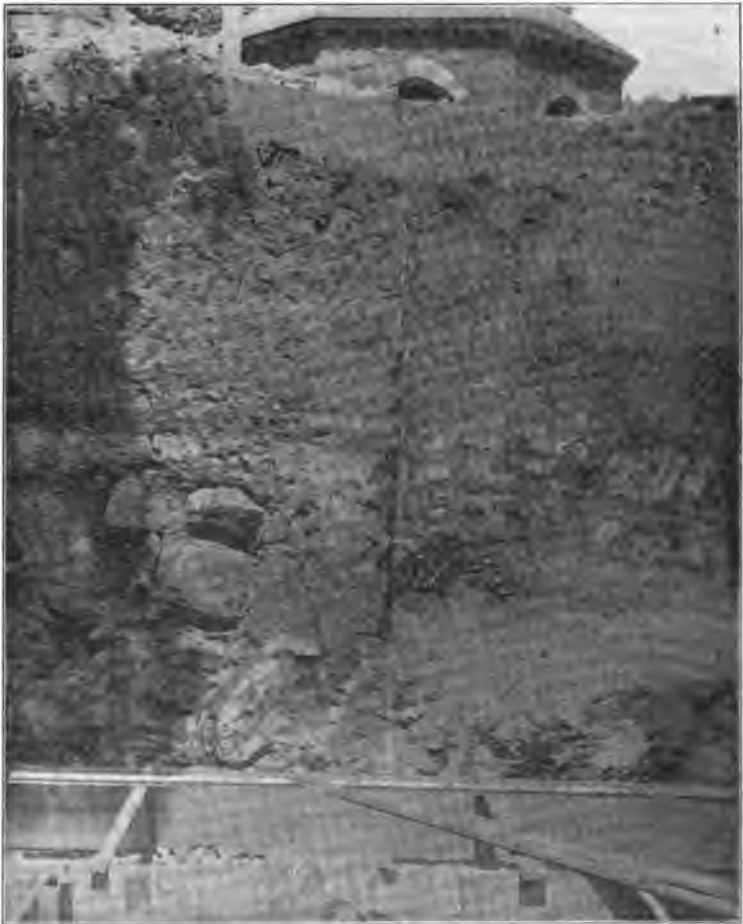
FIG. 34. — Soil originating in place by the decomposition of sandstone
