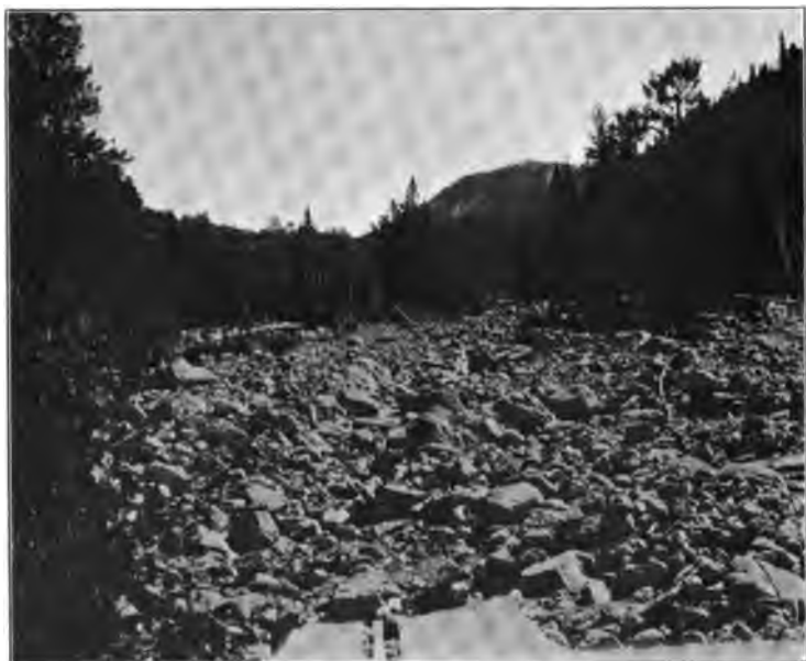
FIG. 91. — Manti Creek, Utah; flood of August, 1901
