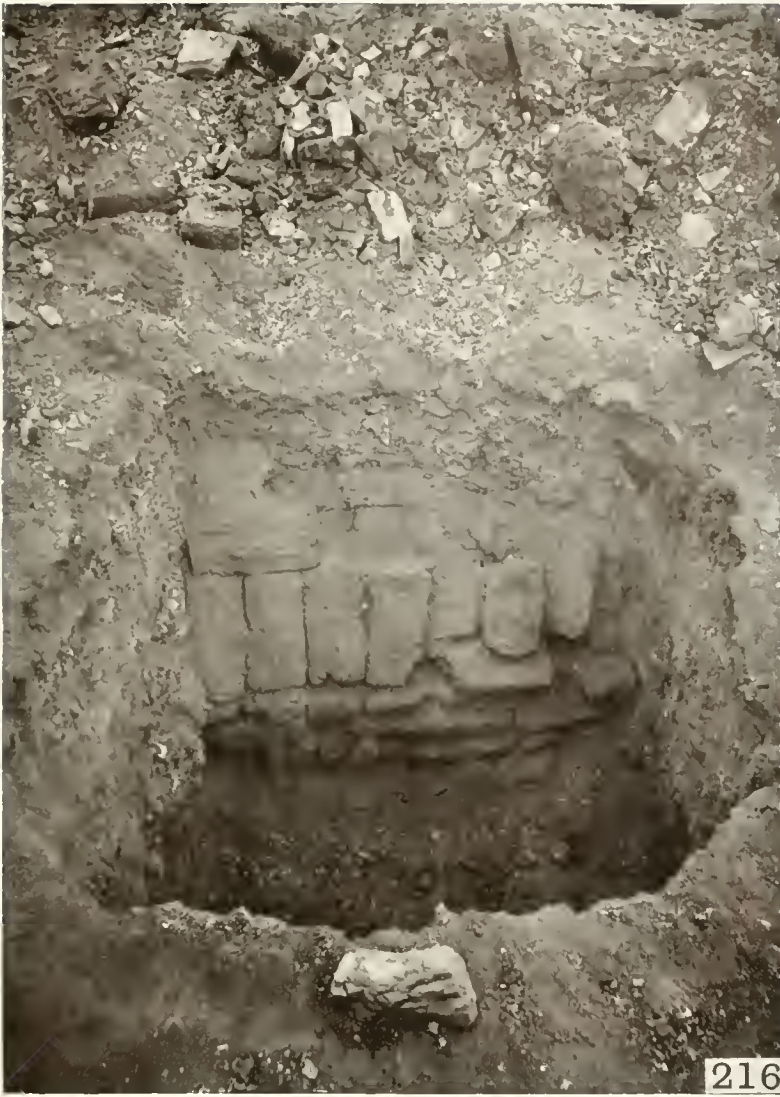
WITH ENTRANCE BRICKED UP.
