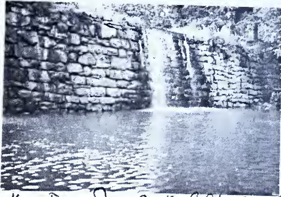
Woodberry Dam on Jones Creek, Powhatan, Co. Va.
